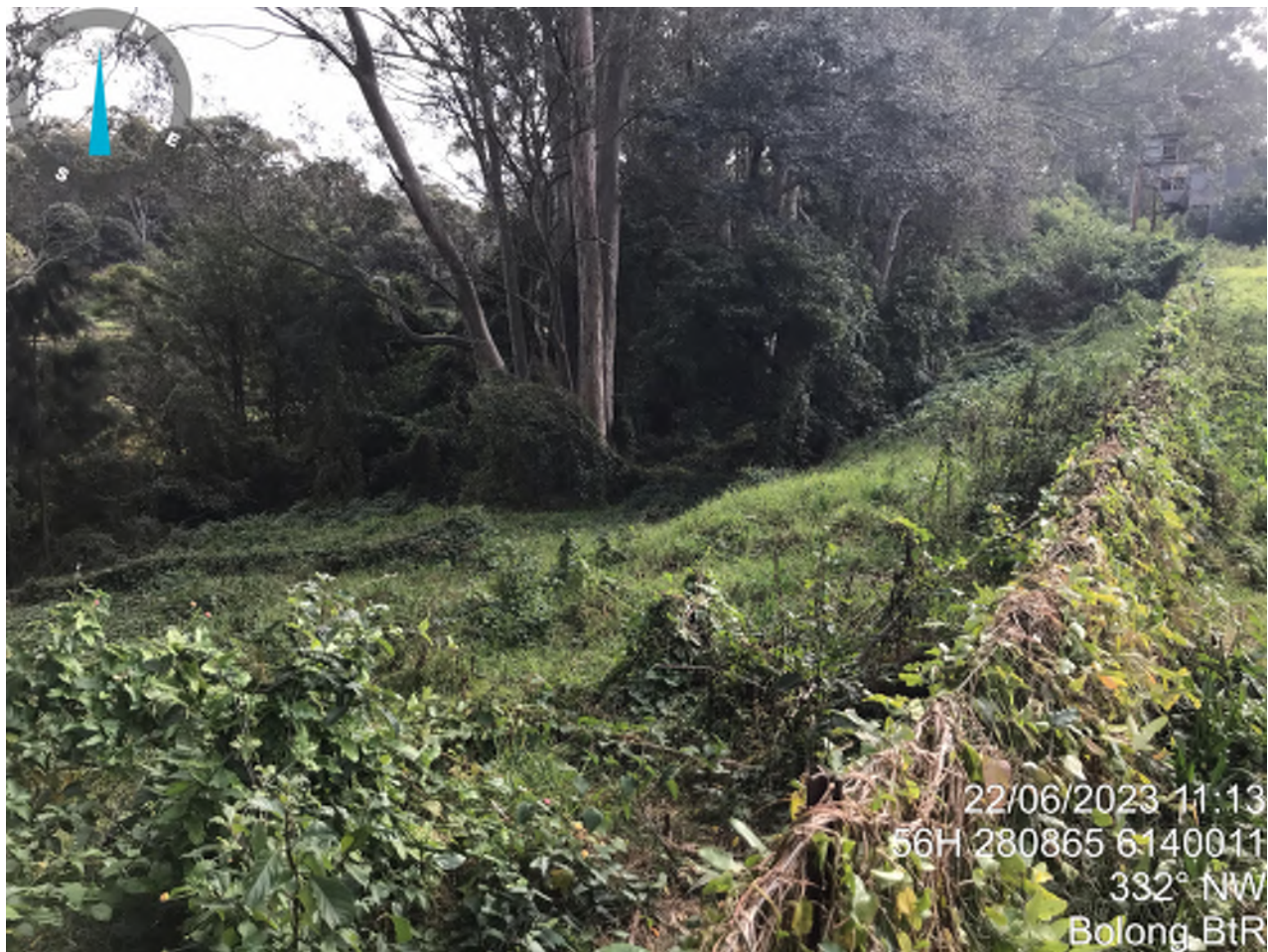
PHOTO P1 - WESTERN SLOPE BANK SLOPING AT ~20 DEGREES
