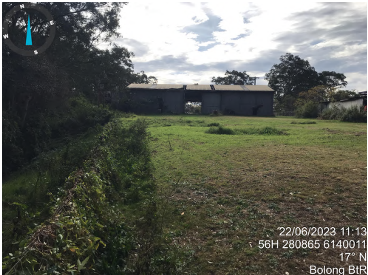
PHOTO P2 - IRREGULAR HUMMOCKY SURFACE INDICATING PRESENCE OF FILL
