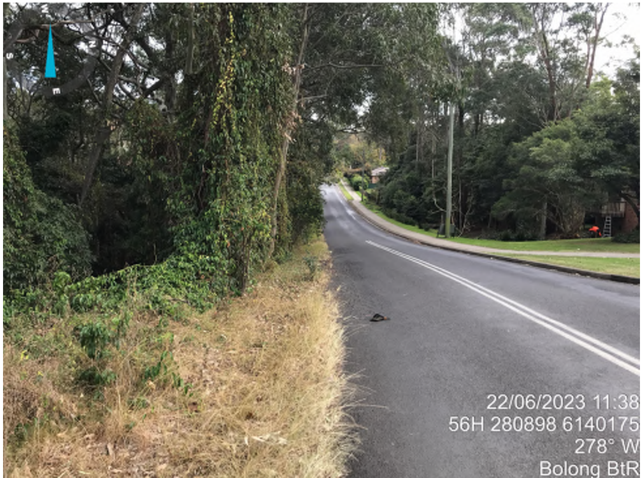
PHOTO P5 - LOOKING WEST TOWARDS SWAMP CROSSING ON BEINDA STREET
